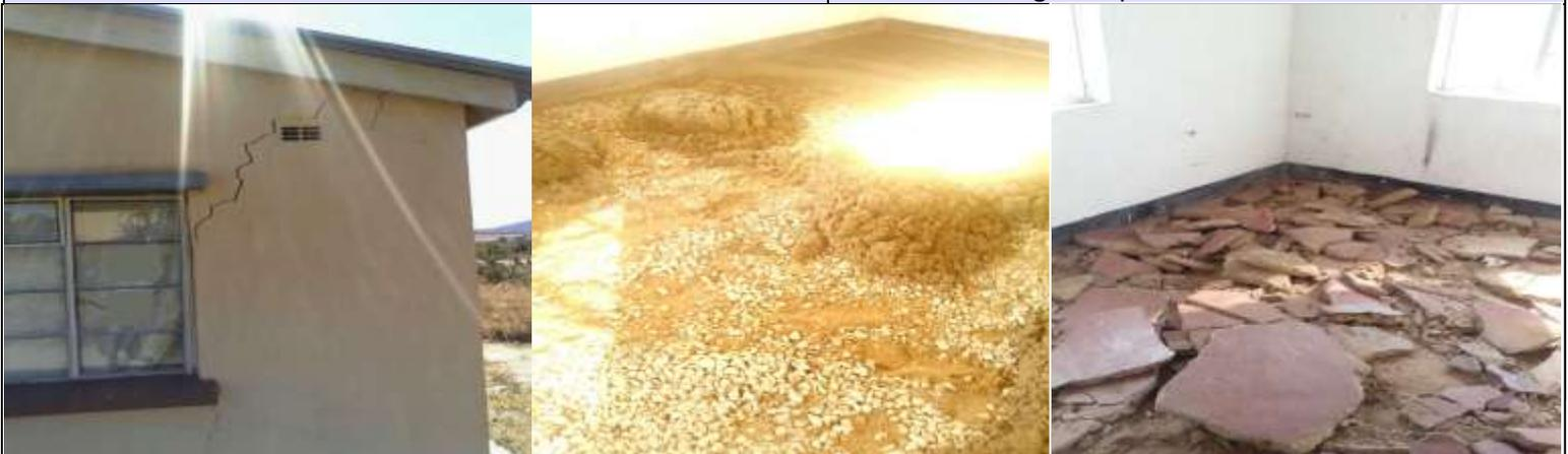
*Poor workmanship at the fast tracked Anjin built Houses at Arda Transau causing walls to crack and floors to disintegrate*
